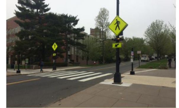
Rectangular Rapid Flashing Beacon
