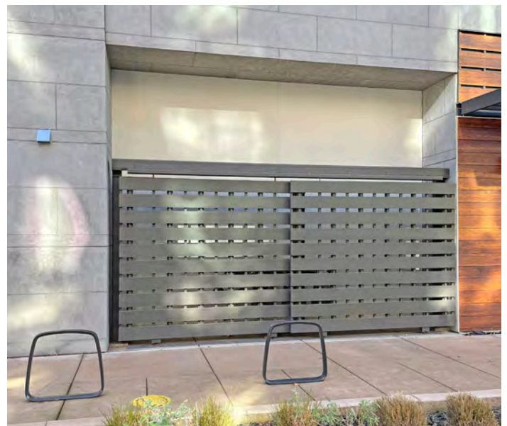
Refuse area with screening from public view.
