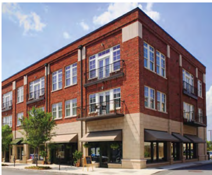
Mixed-use building showing a clearly defined base, middle, and top.
