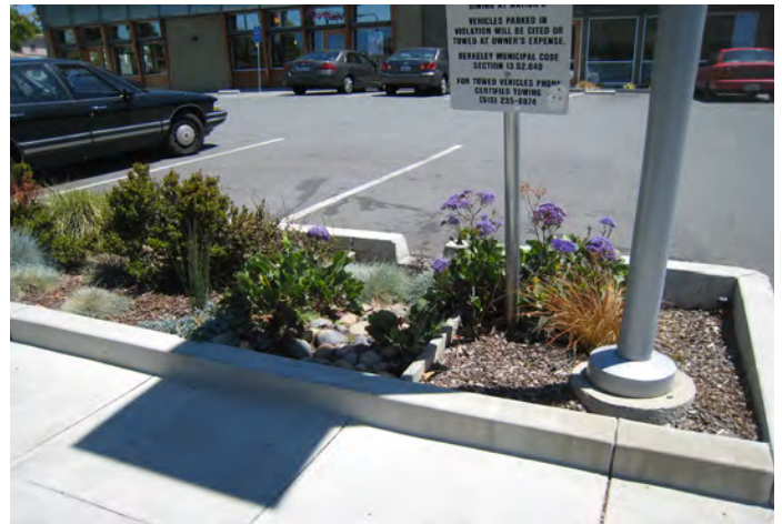
Stormwater bioretention area in parking area.
