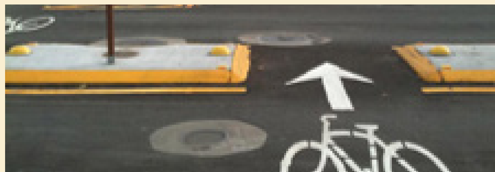
Traffic calming and diversion
