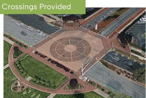
E Hillsdale Boulevard at Central Park Lane Decorative intersection and crossings on all legs
