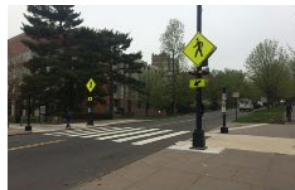
Rectangular rapid flashing beacon and High Visibility crosswalk Source: Federal Highway Administration.
