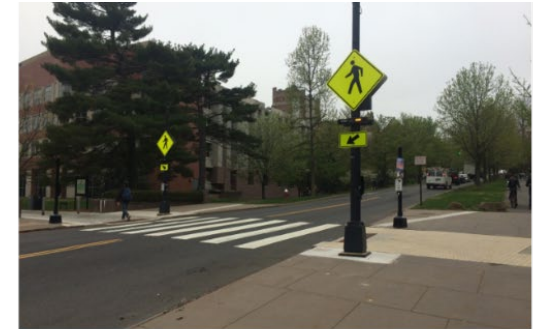
Rectangular rapid flashing beacon and High Visibility crosswalk
