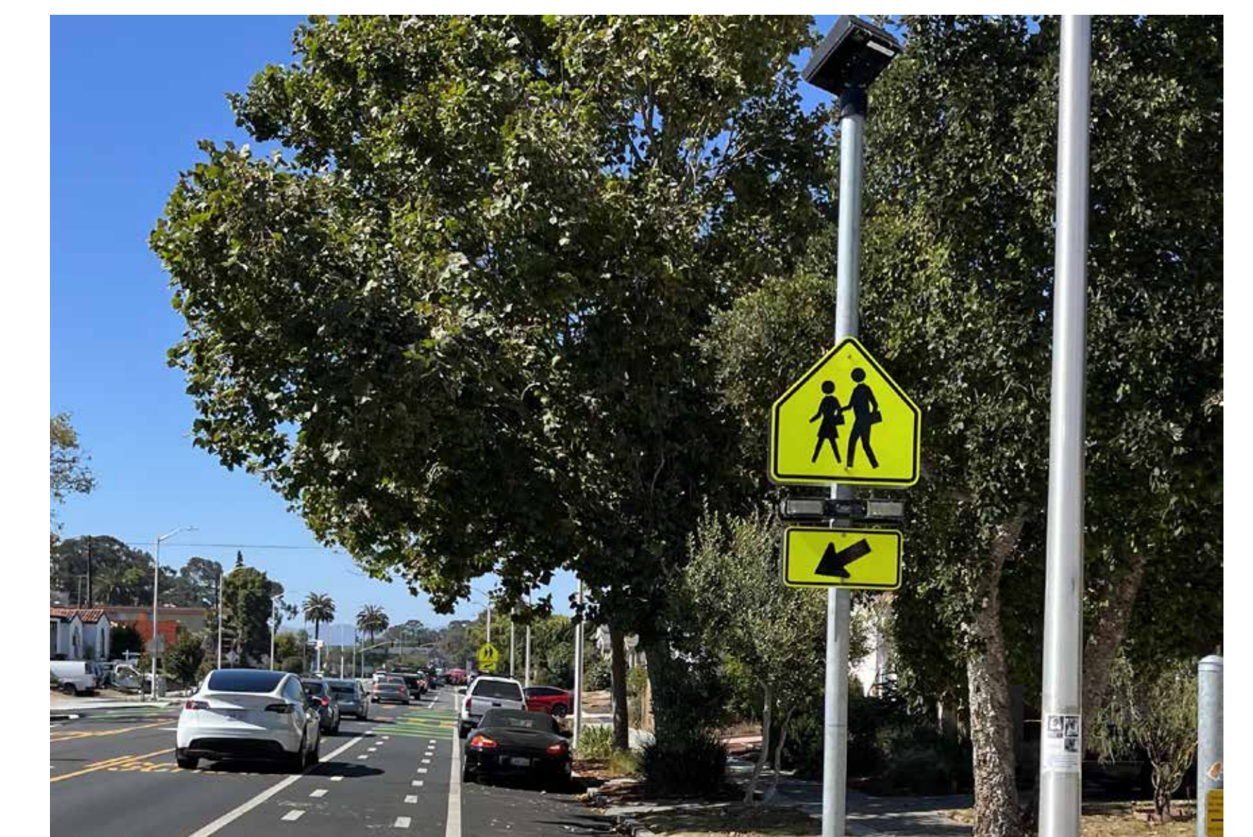
Rectangular Rapid Flashing Beacon and High Visibility Crosswalk
