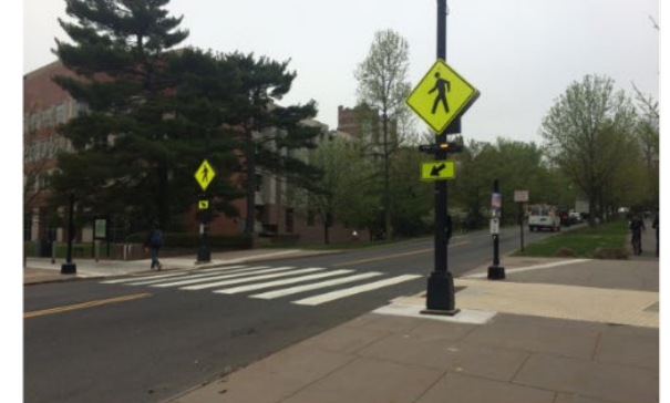
Rectangular Rapid Flashing Beacon
